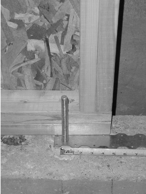
Figure 4.1. End-wall strap before installation.
